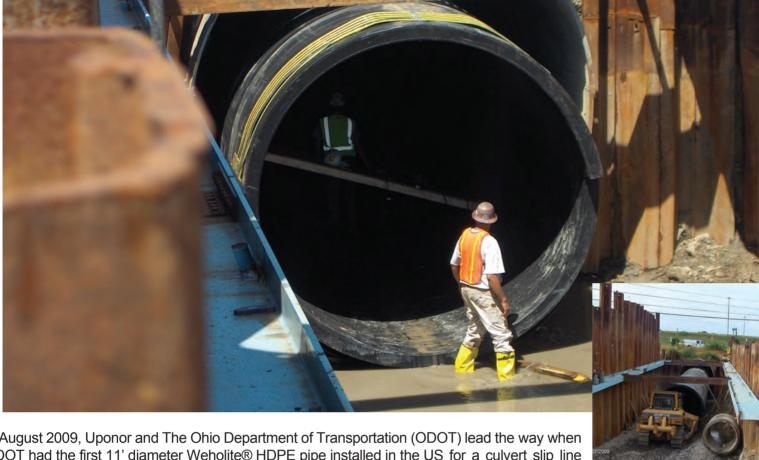
In August 2009, Uponor and The Ohio Department of Transportation (ODOT) lead the way when ODOT had the first 11' diameter Weholite® HDPE pipe installed in the US for a culvert slip line application. The existing 1000' long 15' diameter CMP culvert had been extended an additional 260' with a 10' CMP culvert. The culvert carries a tributary of the Chagrin River under Rte. 2, its interchange ramps and two local streets. There were also nine laterals, including one measuring 72" and one 66".
